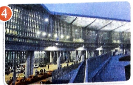
Netaji Subhas Chandra Bose International Airport
